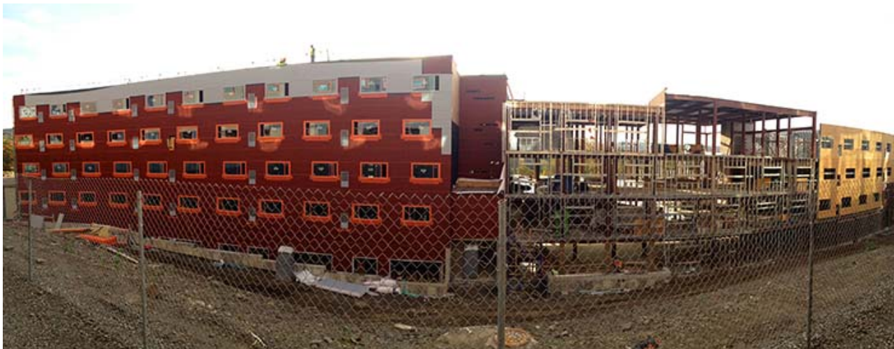
Photo by Excel Engineering, Inc.
